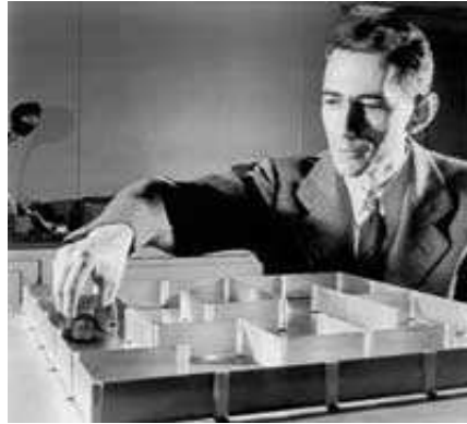
Figure 1.1: Shannons original mouse labyrinth.
